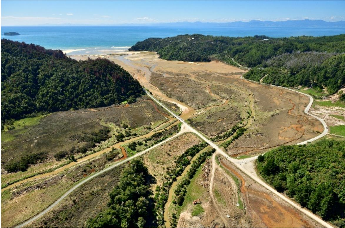
Figure 2.25 Thin debris flow and over bank deposits, lower Holyoake Stream valley and mouth, Otuwhero inlet.
