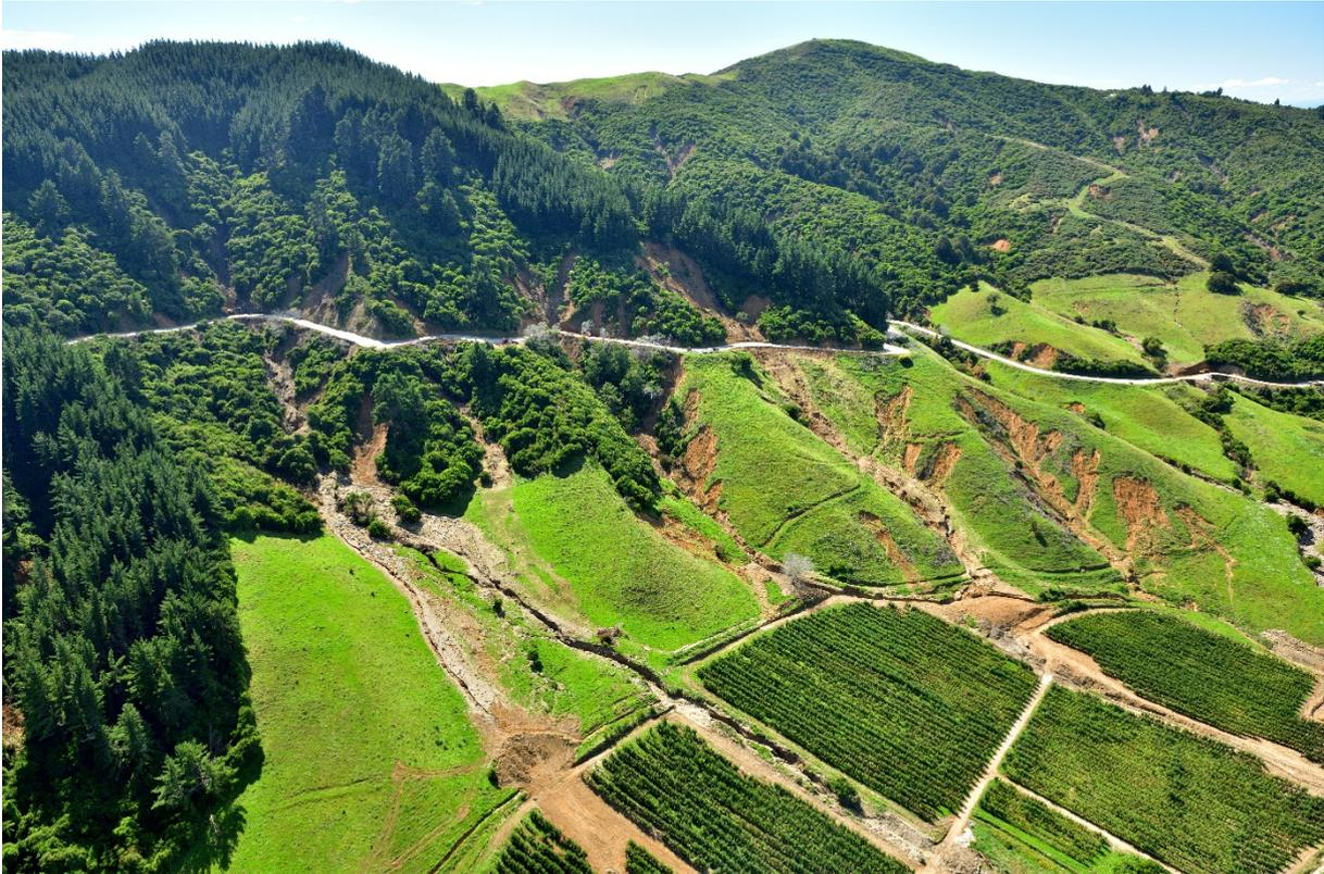
Figure 2.16 Landslides and debris flows badly damaged the Takaka Hill Road on the north side of the Riwaka valley. In some instances, the road was inundated by debris making it impassable. Many of the debris flows had enough power to erode the edge of the roadway, causing wash-outs below the road.
