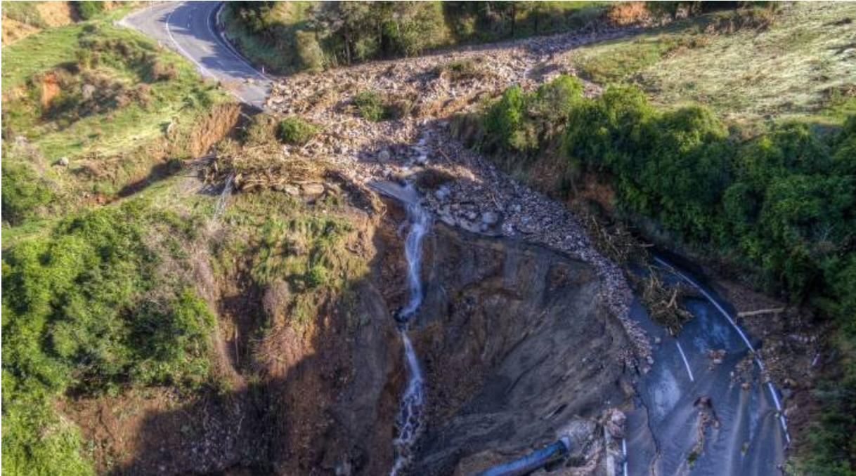
Figure 2.17 A debris flow on the Takaka Hill Road that eroded the edge of the roadway and caused a large washout (Photo: Stuff.co.nz, 22 February 2018).
