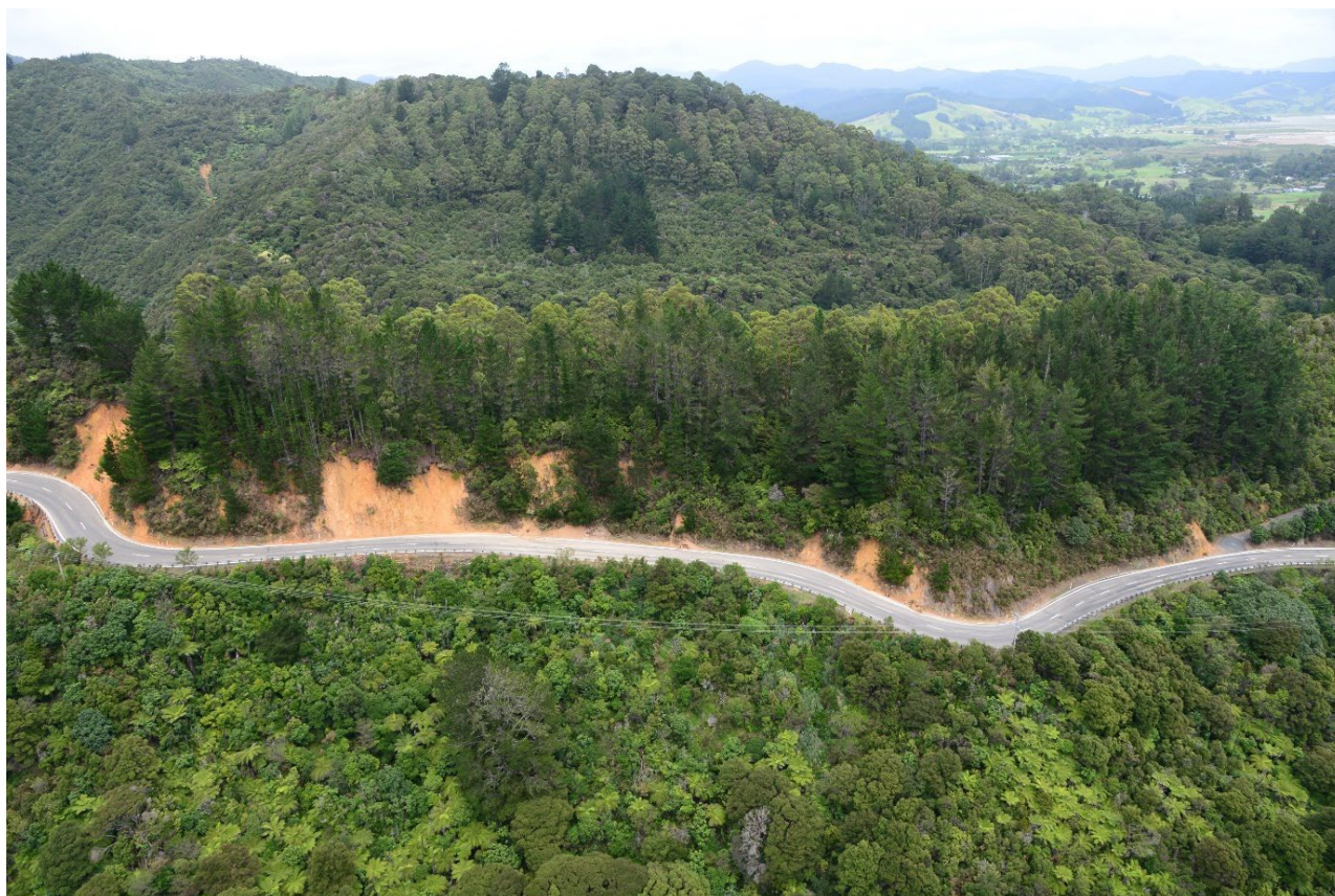
Figure A2.29 Photo DSC_9731: Examples of failures of the cut bank along State Highway 25, Coromandel.
