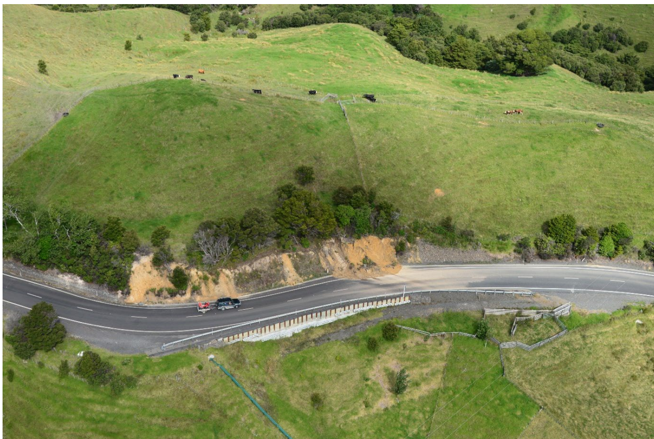
Figure A2.24 Photo DSC_9856: Examples of road-cut failures along State Highway 25, Wilson Bay, Coromandel Range.
