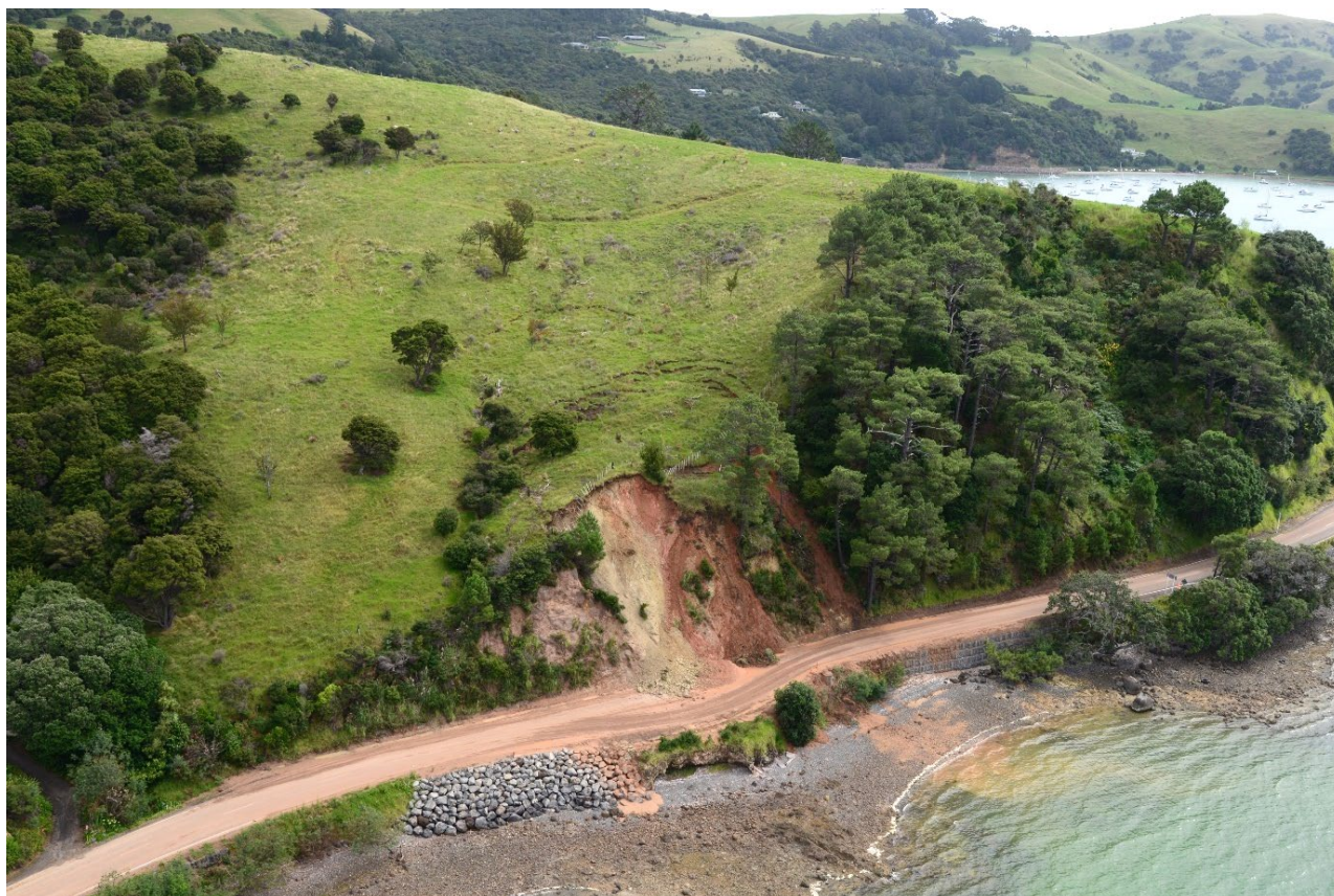
Figure A2.26 Photo DSC_9830: Example of an incipient failure (note the cracks visible in pasture above the debris failure) at Waipapa Bay, Coromandel Harbour.
