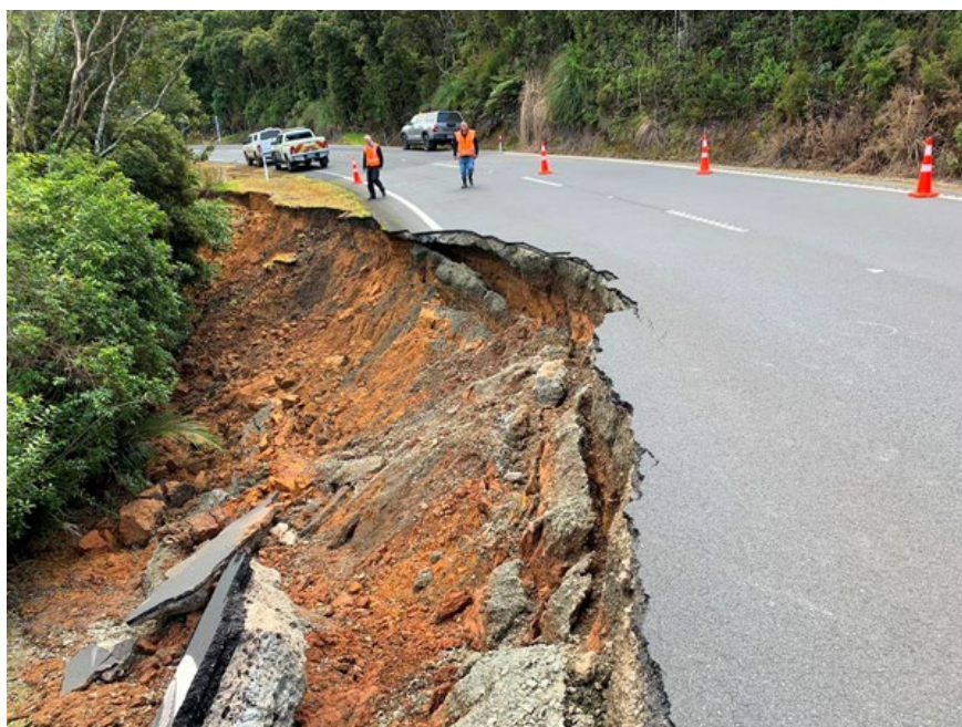
Figure 3.2 One of the landslides (drop-out) affecting State Highway 1 through Mangamuka Gorge (Photo: Waka Kotahi).
