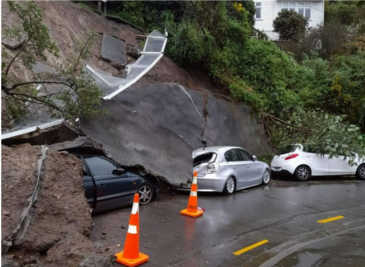
Figure 3.4 A retaining wall collapsed onto cars on Sutherland Crescent in Melrose. (Photo: Mark Remfrey / Wellington Region Emergency Management Office (WREMO) Facebook page).
