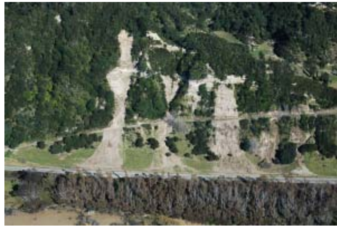
Debris avalanches from the old seacliff, northwest of Matata, at Herepuru Road.
